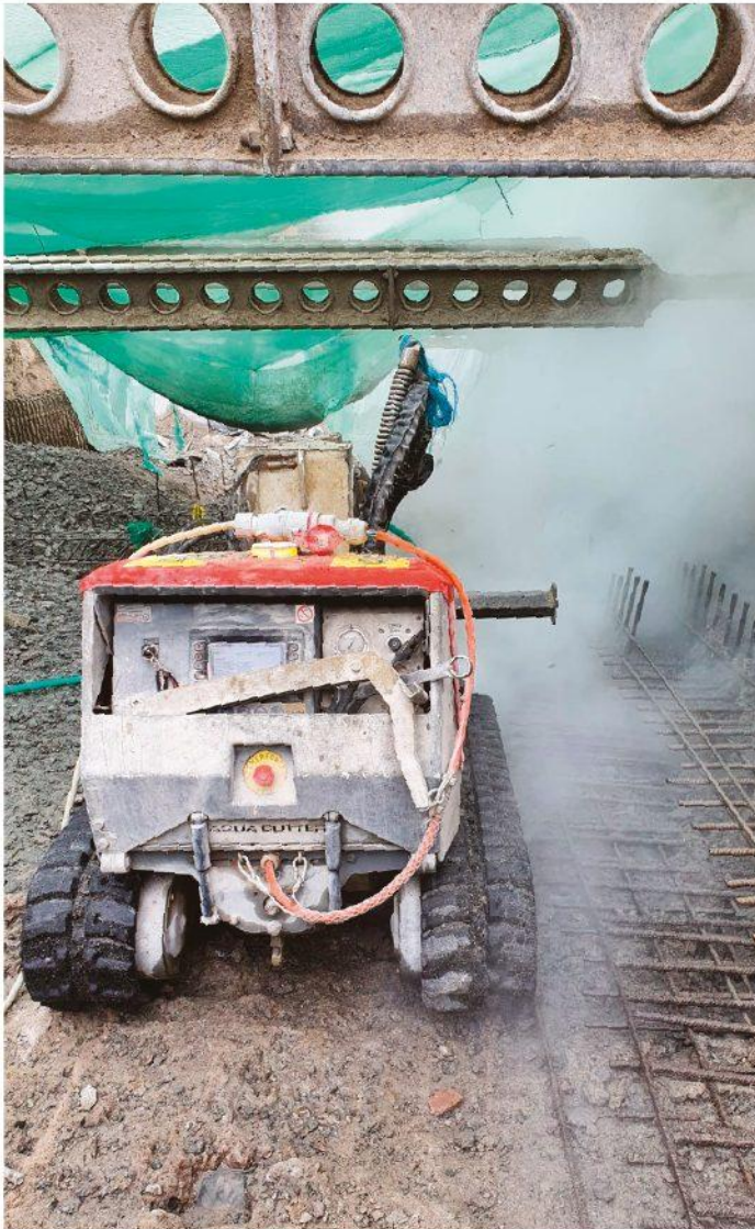
AquaJet system positioned to work safely along the steep sluice.
