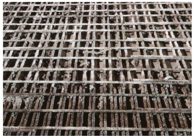
High-pressure water removed deteriorated concrete without impact vibration, leaving the reinforcement intact.
